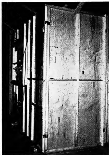
Fig. 3. Rear view of hard flat, corner section, showing structural details.
